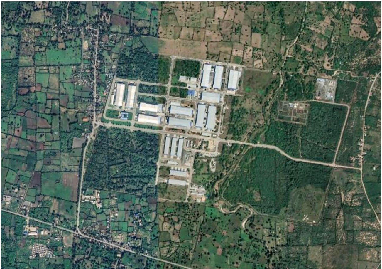
An aerial view of the Caracol Industrial Park, surrounded by farmland.
